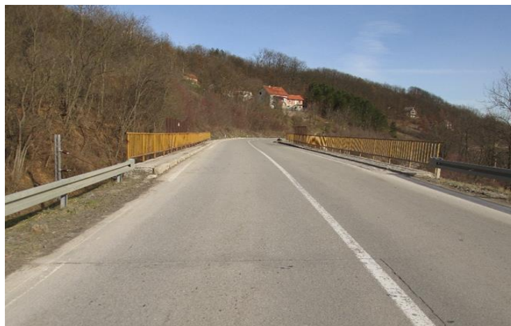
Figure 23. Overpass at Belgrade-Bar railway near Kosjeric
