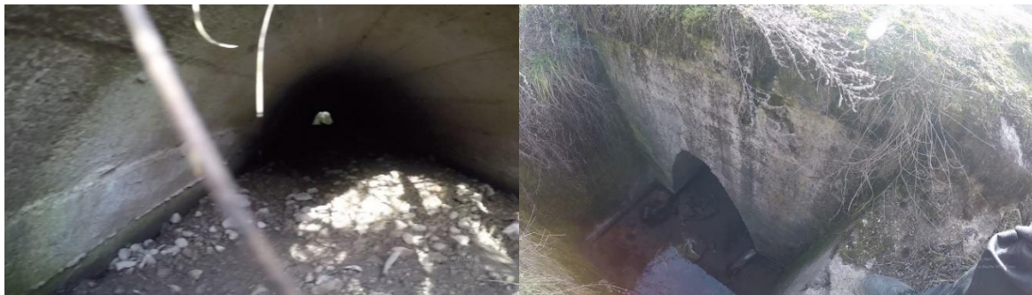
Figure 32. Arched culvert at ~ km184+881
