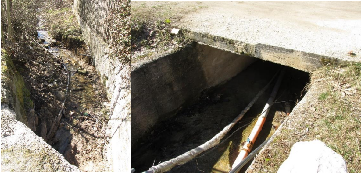
Figure 34. Slab culvert at ~ km 188+750
