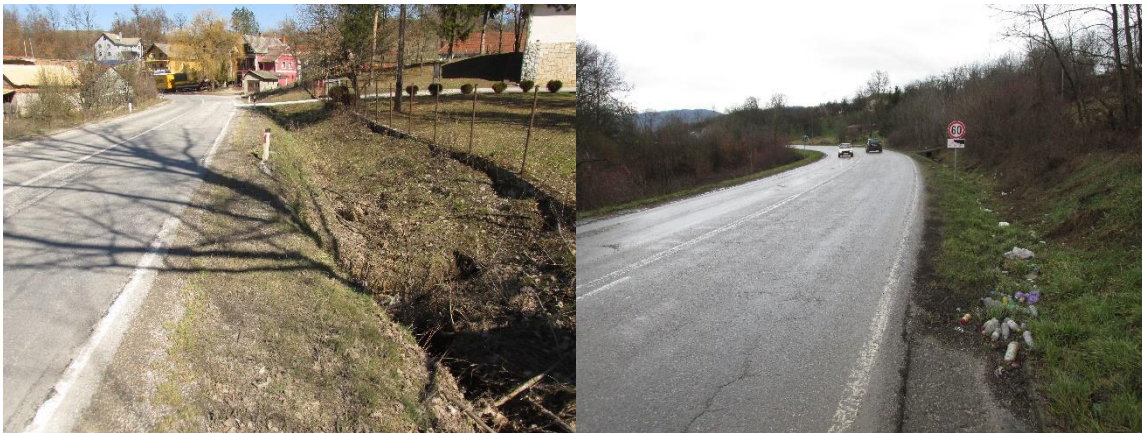
Figure 13. Canals on the observed road section
