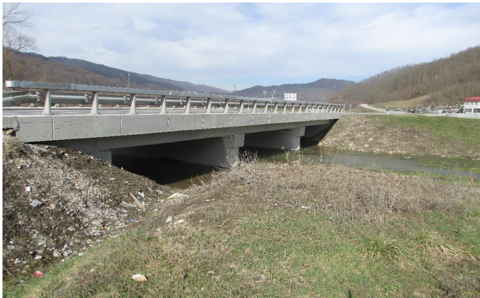
Figure 29. The Bridge over Dobrinjska River at km 198+247
