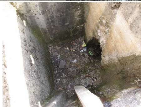
Figure 33. Combined culvert at ~ km 185+413
