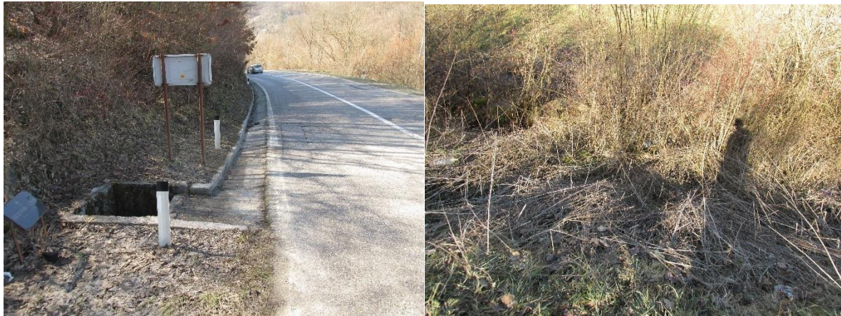
Figure 30. The inlet structure of pipe culvert that collects runoff from gutter, the outlet structure of culvert overgrown with vegetation
