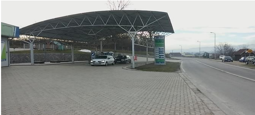
Figure 20. Petrol station „Gaga petrol“ at ~ km 204+900
