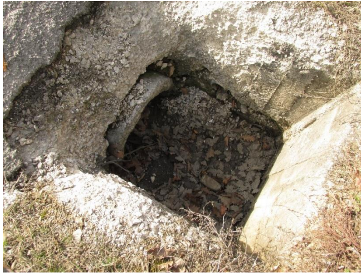
Figure 31. An example of inlet structure of the pipe culvert at ~ km 192+612
