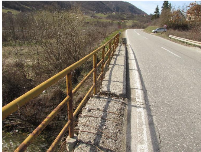
Figure 10. The Bridge over Nenadkovice River at ~ km 188+094
